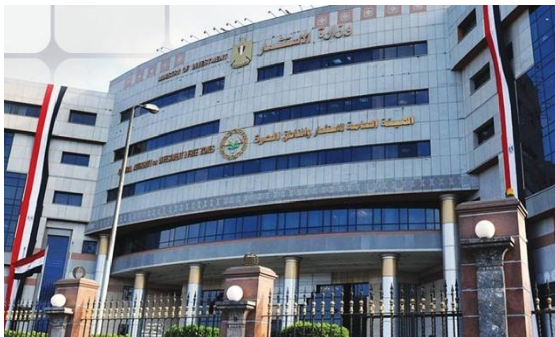
General Authority for Investment headquarters- press photo
